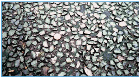
Close up of tarmac worn smooth after 8 years of heavy use
